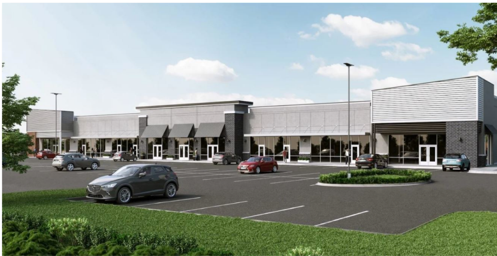
Shopping Center. New Construction with Contemporary Design 1,024' of frontage on FM 1488.
